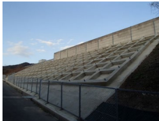
(盛土のり面補強の状況)
